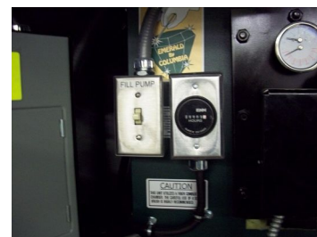
Fill Pump Switch and Hour Meter
